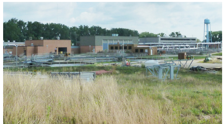
The City of Grand Rapids Waste Water Treatment Plant, located across the Grand River from the site (see Figure 3), receives electricity from Consumers Energy.
