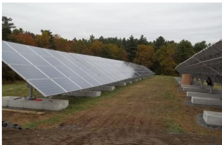
A 2.1 MW solar PV project in place at the East Hampton Landfill in western Massachusetts is an example of a solar project designed for compatibility with an existing remedy. Solar PV arrays are mounted on ballasted foundations that rest on top of the landfill cover system (above left); the configuration of the site’s solar PV network is designed to allow for access to existing remedy components, such as landfill gas collection and ground water monitoring wells (above right). Image source: Borego Solar
