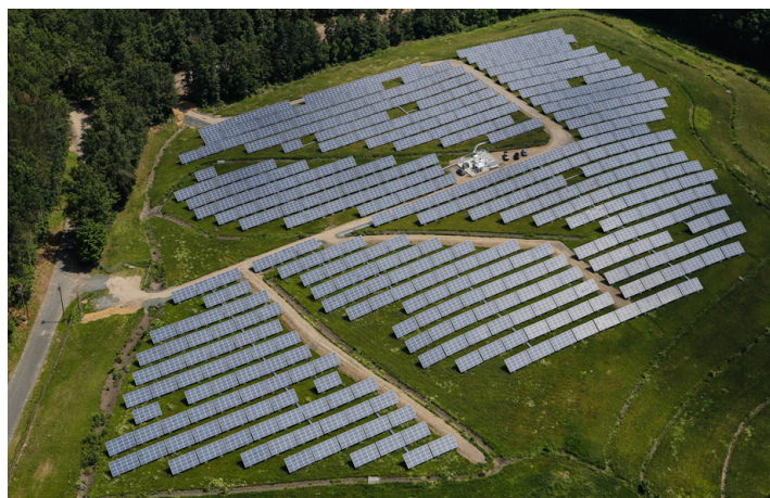
A 2.1 MW solar PV project in place at the East Hampton Landfill in western Massachusetts is an example of a solar project designed for compatibility with an existing remedy. Solar PV arrays are mounted on ballasted foundations that rest on top of the landfill cover system (above left); the configuration of the site’s solar PV network is designed to allow for access to existing remedy components, such as landfill gas collection and ground water monitoring wells (above right). Image source: Borego Solar
