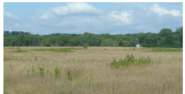
Capped area in Western Landfill Unit
