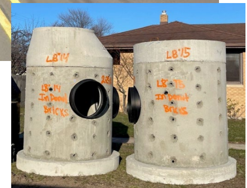
Leaching Basins Prior to Installation
