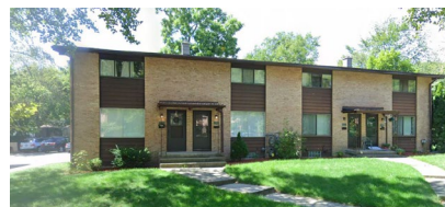
Mid-20th Century townhouses in the Creston Neighborhood, grouped in fours, fronting on a street with parking in the rear.
