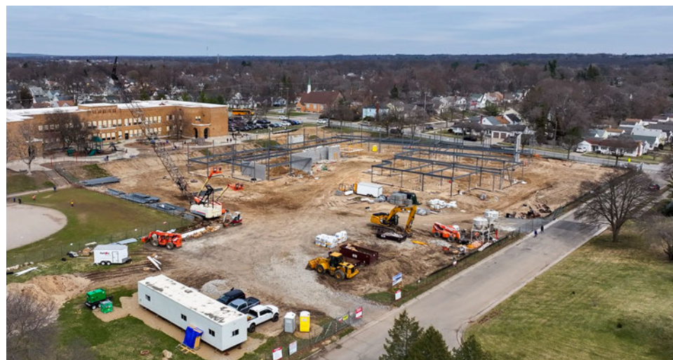
Construction continued through the winter on a new, state-of-the-art elementary school on the site of Aberdeen Academy.
