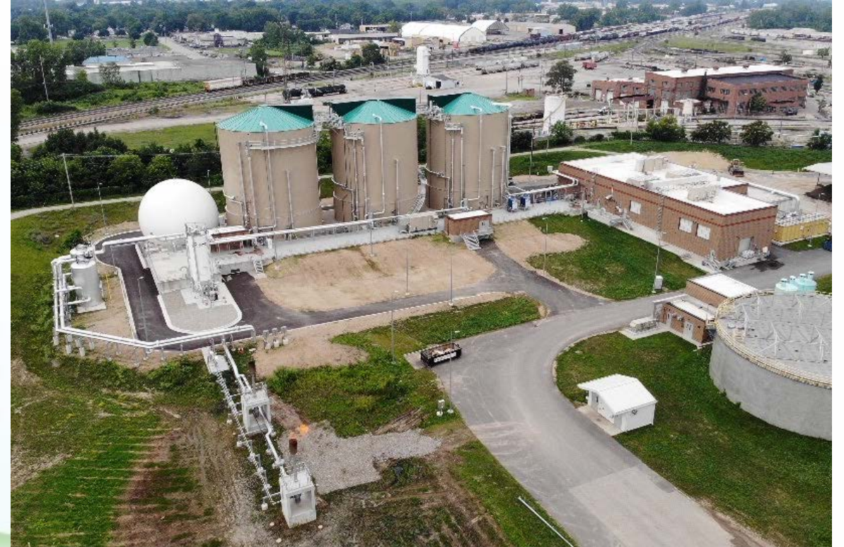
Biodigester and related projects at the WRRF
