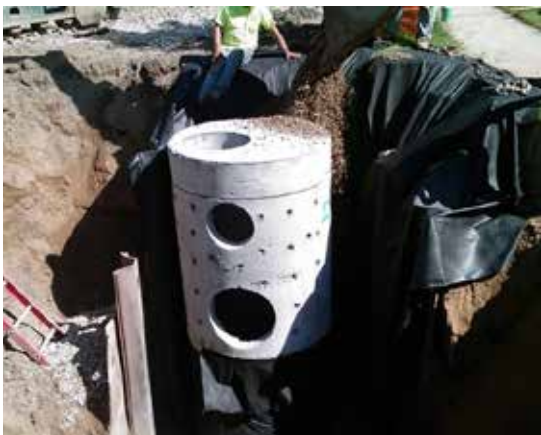
Figure 25. The City has installed a number of infiltration basins around town to capture stormwater near where it falls to help it slowly seep back into the ground. Photo: Grand Rapids Environmental Services Department
