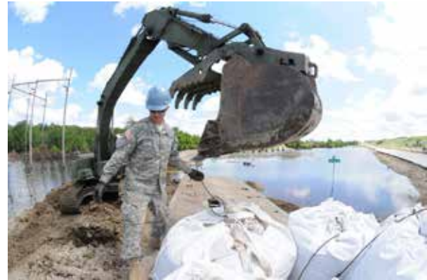
Figure 21. Horizontal Engineering Company works with the Minnesota Army National Guard to repair a levee. Photo: Sgt. First Class Daniel Ewer, U.S. Army
