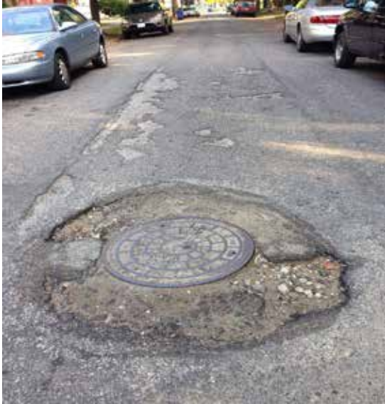
Figure 15. Periods of high temperatures soften and expand roadway materials, creating ruts, which are exacerbated by vehicles to create potholes. Photo: Nicholas Occhipinti
